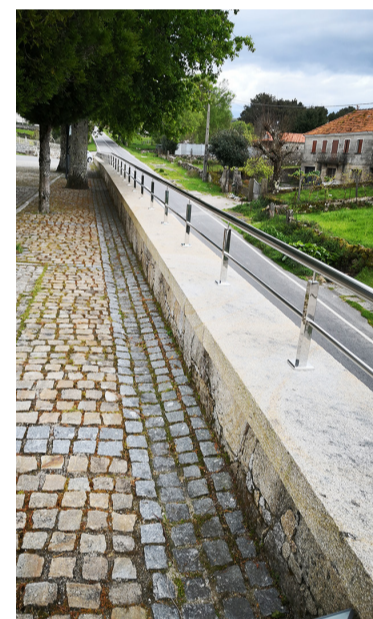
Grade do muro
